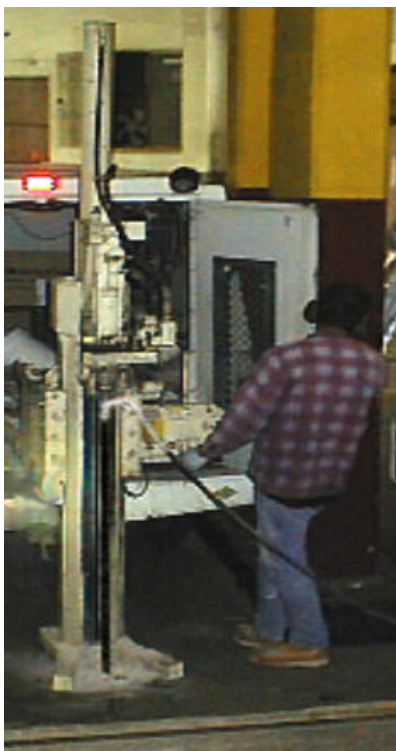
Injecting hydrogen peroxide through the drill rod of a direct push rig.
